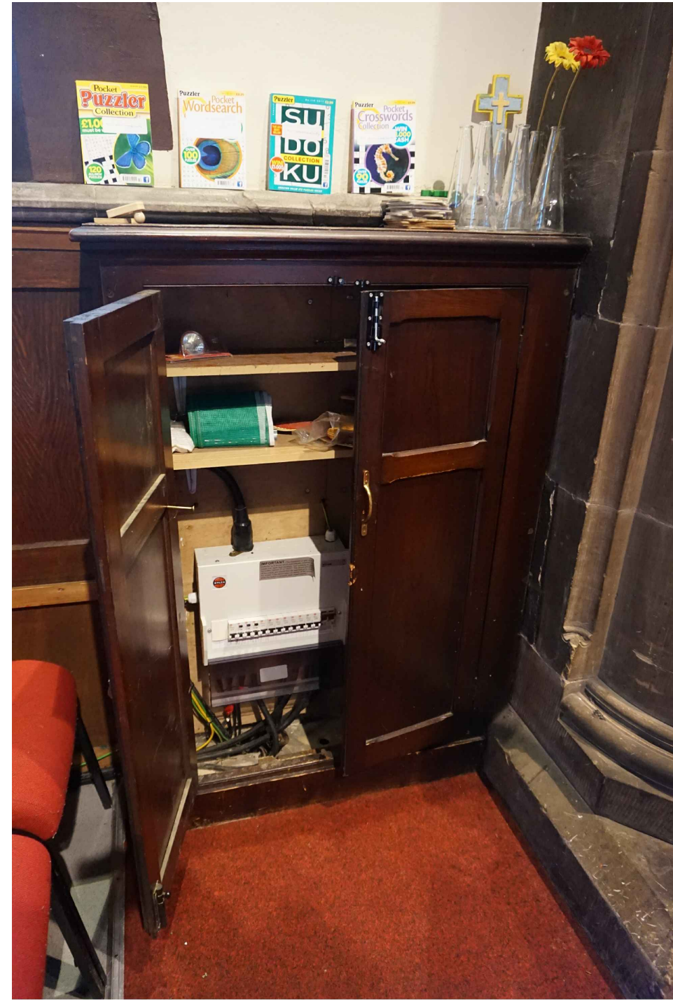
Photograph 05 Existing fuse board cupboard
